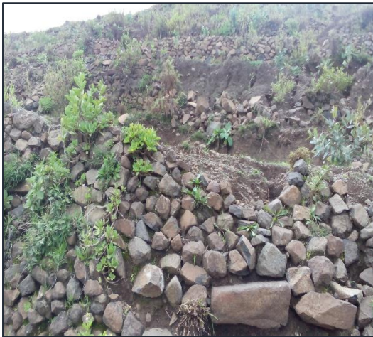
Fig. 4. Collapse of terraces due to single line stone placement, no buffer zone and not support with biological SWC practices
