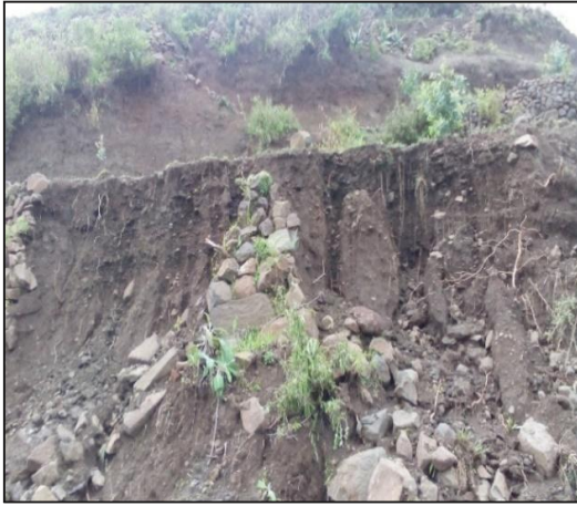
Fig. 4. Collapse of terraces due to steep slope and fragile soil
