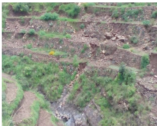
Fig. 6. Collapse of the terrace due to not recommendable slope
