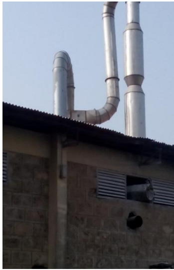
Plate 1b. Positive Single Cyclone System
