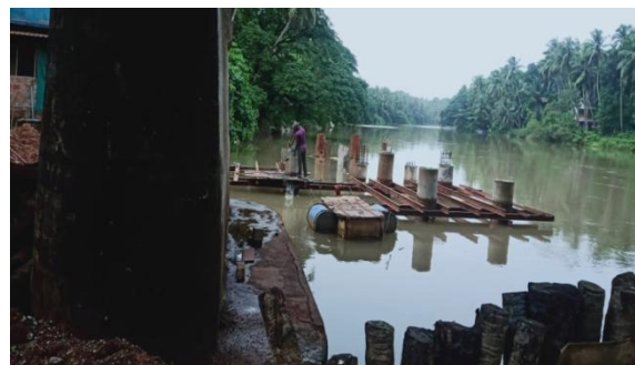
Image 5. Showing new bridge construction at Mambaram
