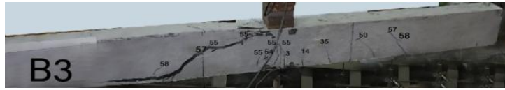
a) Cracking Patterns for Beam (B3) [EXP]
