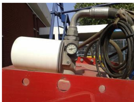
Figure 8. Pressure gauge for checking hydraulic oil pressure
